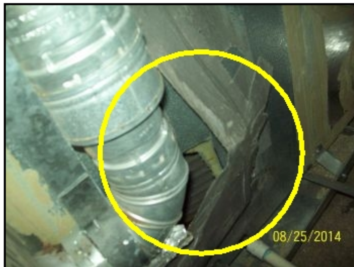
Air leaking at plenum.
