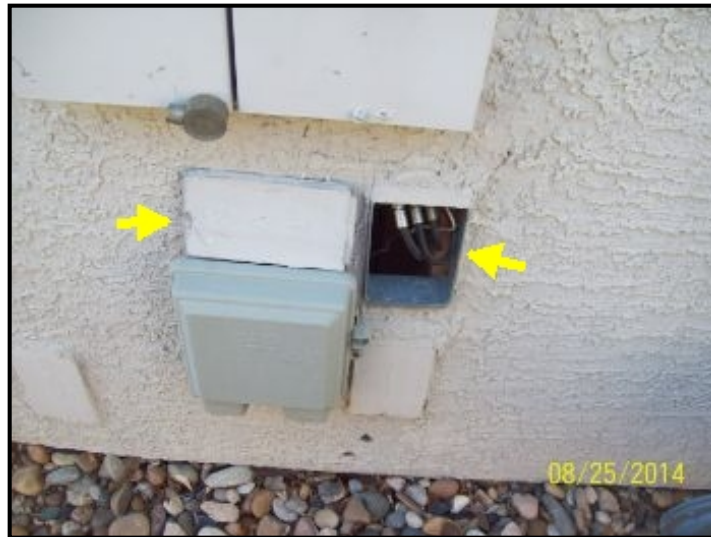
Observed cover to exterior main panel not installed
