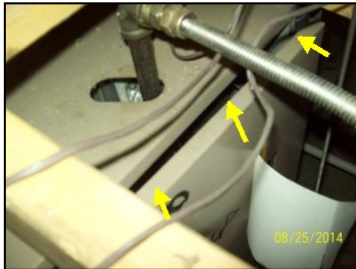
Observed furnace cover loose at unit
