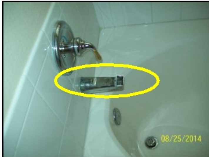
Loose tub fill spout.
