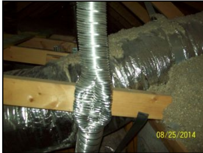
Exhaust fan duct in attic bent
