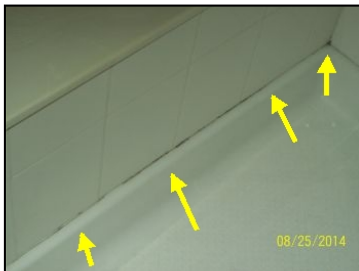
RegROUT tub/shower area as required
