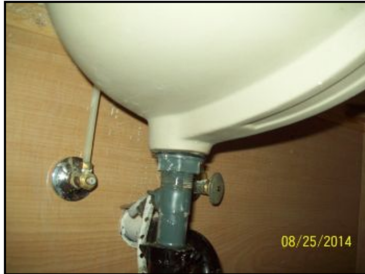
Drain line leaks under sink.
